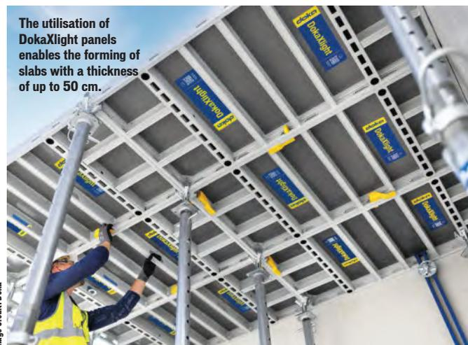
The utilisation of DokaXlight panels enables the forming of slabs with a thickness of up to 50 cm.
