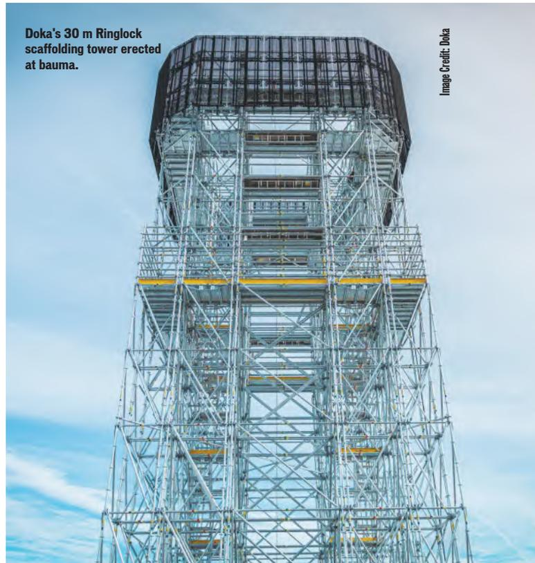
Doka's 30 m Ringlock scaffolding tower erected at bauma.
