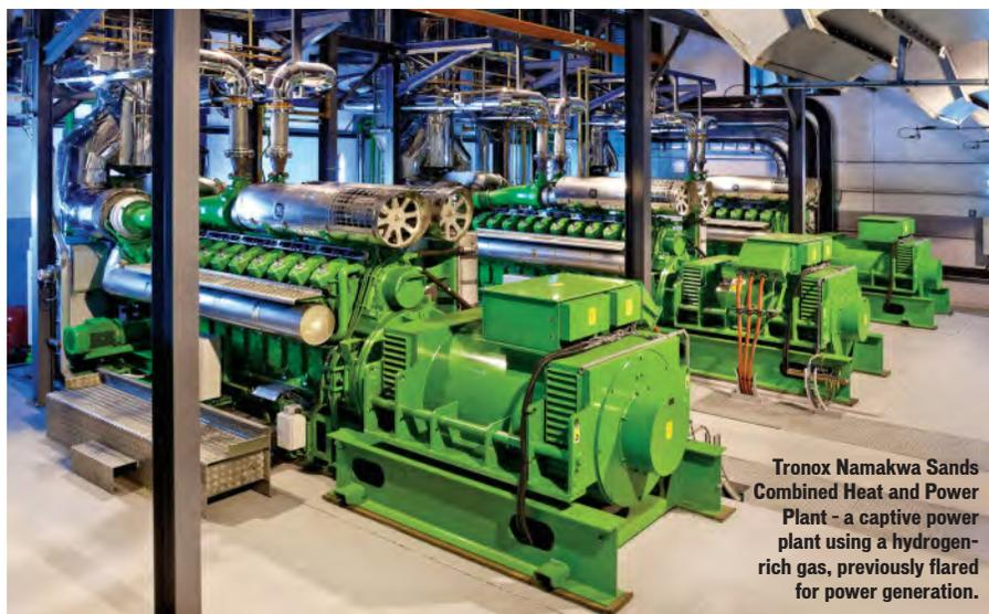
Tronox Namakwa Sands Combined Heat and Power Plant - a captive power plant using a hydrogen-rich gas, previously flared for power generation.
