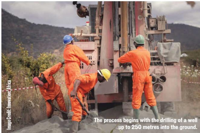
The process begins with the drilling of a well up to 250 metres into the ground.
