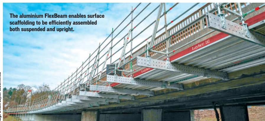
The aluminium FlexBeam enables surface scaffolding to be efficiently assembled both suspended and upright.
