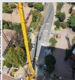
Safe lifting plans are key to a safe work area.
