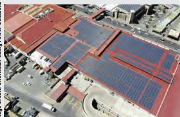
The rooftop photovoltaic system was completed in eight weeks.
