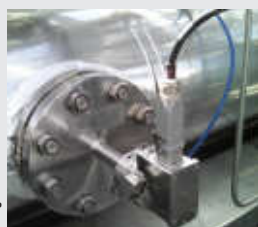
Endress+Hauser Raman probe in a bunker ship.
