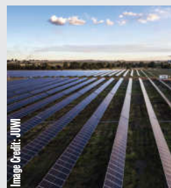
The Evander Mines solar photovoltaic plant.
