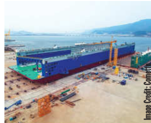
A total of 380 modular axle lines of Cometto MSPE were assembled for the task.
