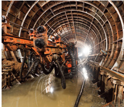
The construction of the diversion tunnels is around 85% complete.
