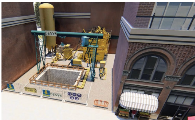
The minimally invasive BAUER Cube System reduces the surface impact of cutting sites to a minimum.
