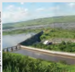
The dam site is on the largest waterfall in the world by volume, the Inga Falls.
