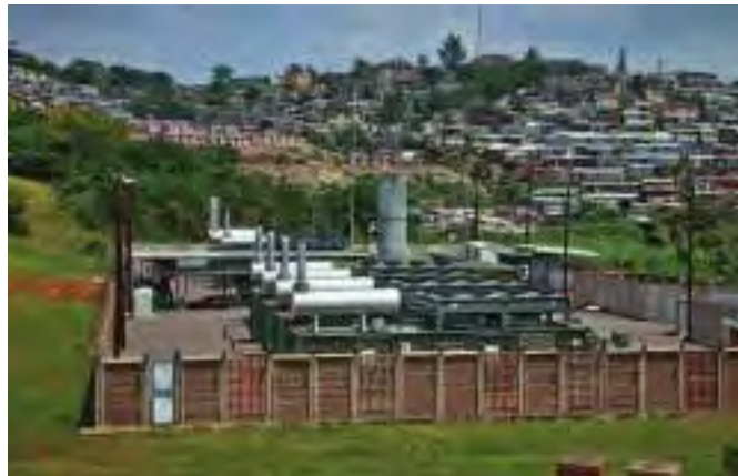
A landfill gas power station using GE's Jenbacher engines at Bisasar Road, Durban, South Africa. (Source: Clarke Energy)
