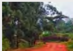
Road projects include Uganda's Entebbe and Kampala-Jinja Expressways. (Source: Adobe Stock)
