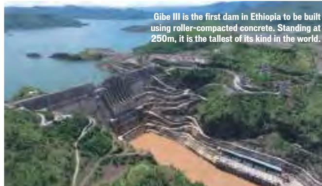
Gibe III is the first dam in Ethiopia to be built using roller-compacted concrete. Standing at 250m, it is the tallest of its kind in the world.
