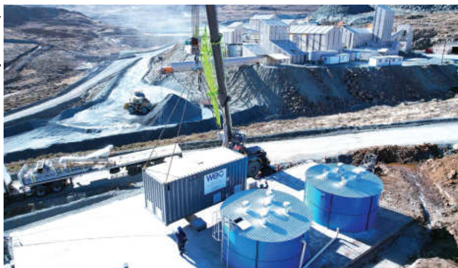
Containerised, modular design of the treatment plant makes for faster installation.
