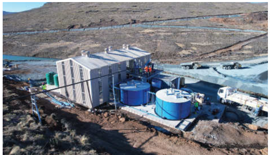
The facility housing the bioreactor on the left ensures that the temperature remains at optimum levels for biological growth.
