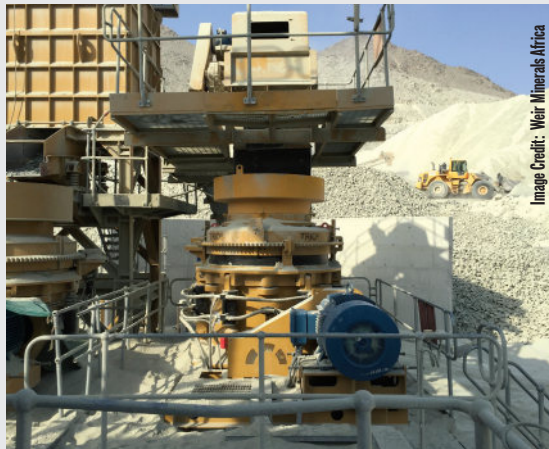
The Trio TP 360 cone crusher installed at an operation in Oman.
