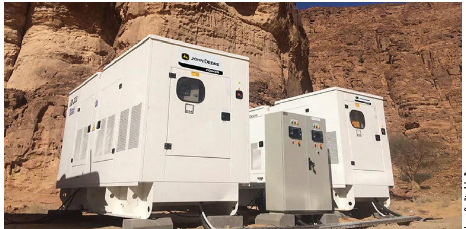
The Tantora project included 33 generators with John Deere engines providing a total capacity of 7.0 mVA.
