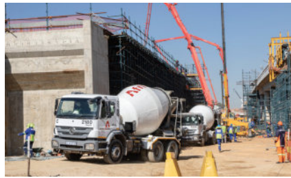
AfriSam dedicated between 14 to 17 trucks to the job of servicing WBHO's concrete pumps during the large continuous pours of around 550 m 3 each.
