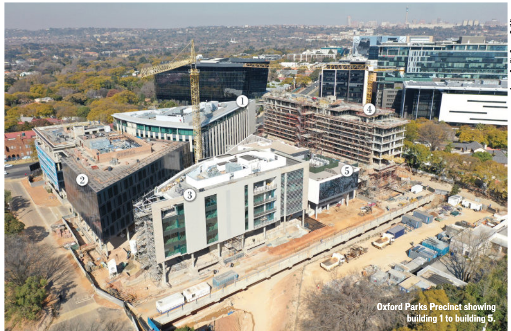
Image Credit: Concor Buildings
