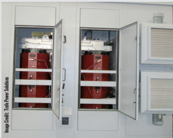
A 3,000kVA dry-type transformer with an IP54 enclosure for a coal mine application.
