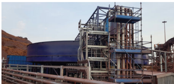
FLSmidth bolted thickeners were selected for a coal plant in Mozambique.
