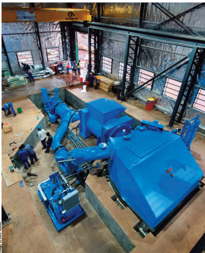
A 3.0MW Turgo turbine has been installed in the Mulosa River project.
