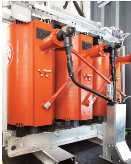
1250kVA cast resin transformer installed inside modular substation.
