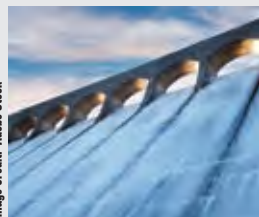
The Ruzizi IV hydropower plant will supply 287MW of electricity.
