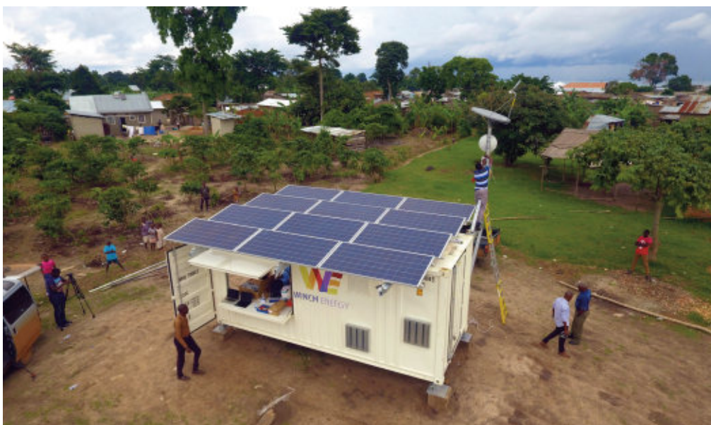
Winch Energy is installing its proprietary unit, the Remote Power Unit, at a number of localised mini-grid projects across Africa.
