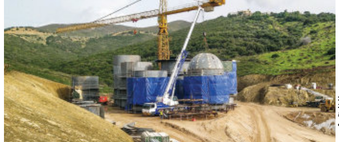
Expansion of a LPG gas tank terminal for Afriquia Gaz with the used LTM 1070-4.2.
