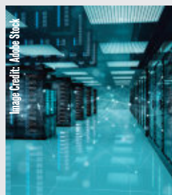
MENA contributes to 2% of the worldwide data centre market.
