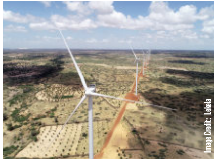
The battery will be located at Lekela's 158.7MW Parc Eolien Taiba N'Diaye (PETN) project.
