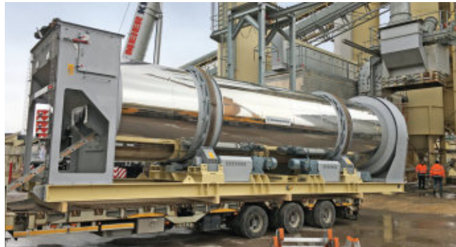
Teamwork: low-loaders transport the new dryer drum to its final position. The Guggenberger crew and the Benninghoven fitters complement one another perfectly in this process.
