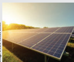
Orange is deploying solar solutions and the latest generation batteries.
