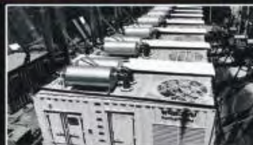
High Voltage 6.3MW Power Plant - Thailand
