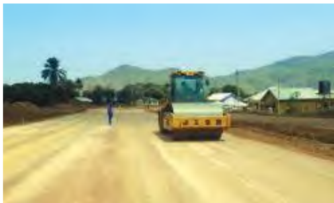
Compaction of the Mbinga-Mbamba road in Tanzania.
