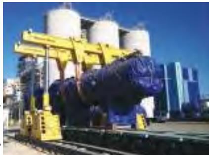
Enerpac SL400 gantry delivers high pressure heaters at Safi coal-fired power plant.
