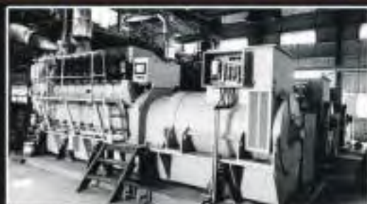
Yaboki-Lac Assal HFO 4.8MW Power Plant - Djibouti
