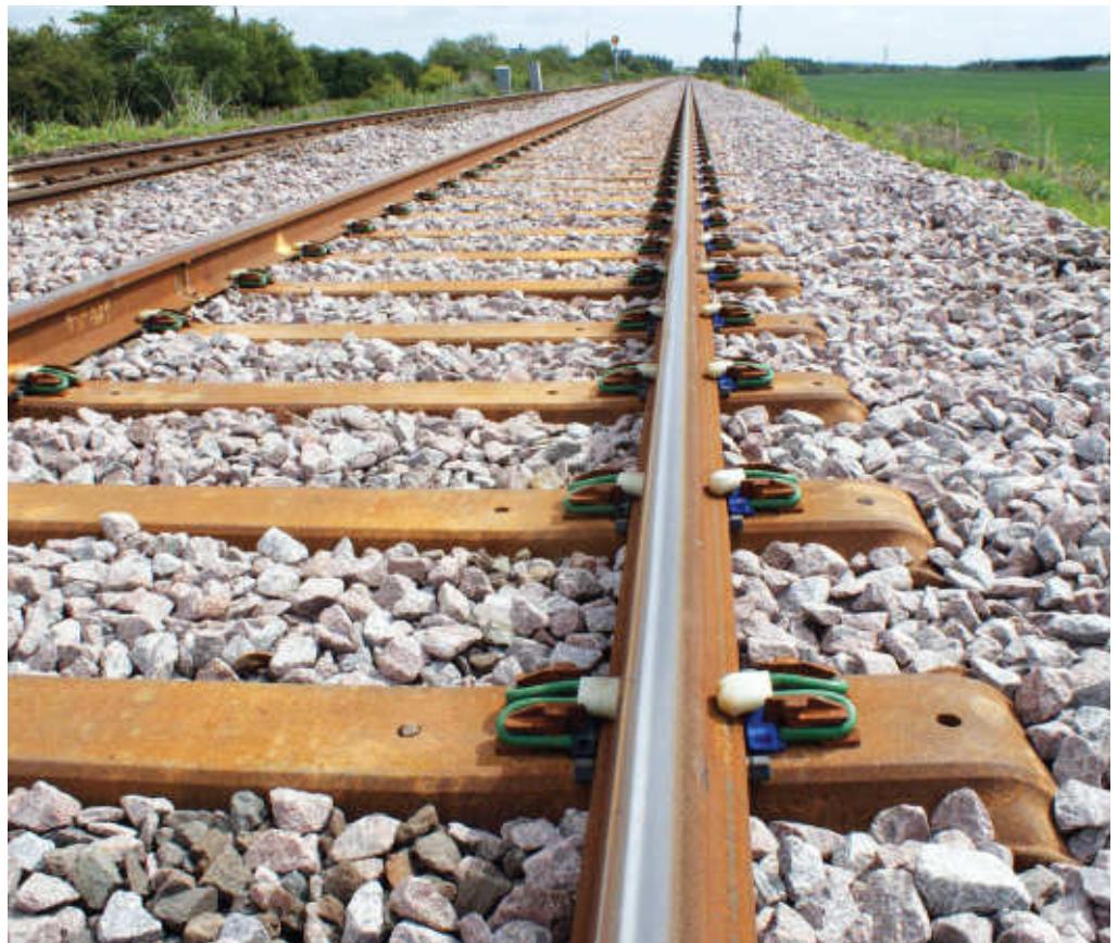
Steel sleepers have tangible advantages over alternatives such as wood and concrete.
