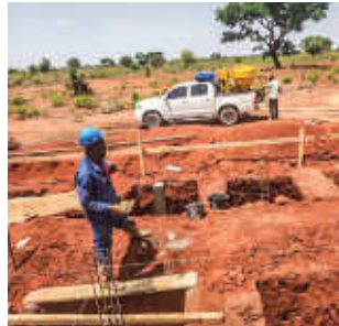
Workers from Setra building the foundations for a water tower.
