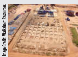
Installation of previously delivered mechanical equipment is progressing well.
