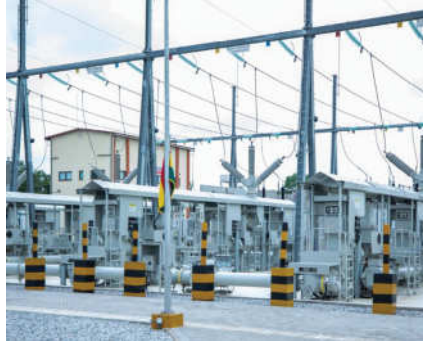
The Kasoa BSP is a 435MVA gas-insulated power substation that will serve 250,000 ECG customers.
