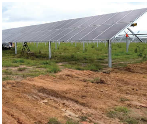
Construction of a solar PV plant in Malawi.
