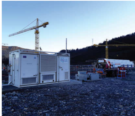
The ACCIONA hydrogen crane.
