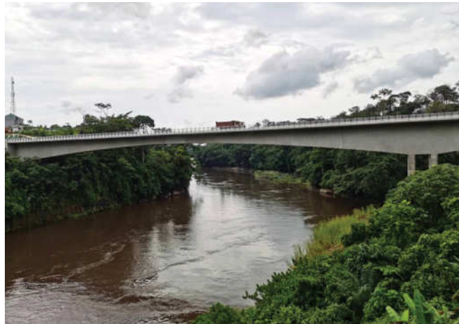
A bridge on the Enugu Bamenda road project.
