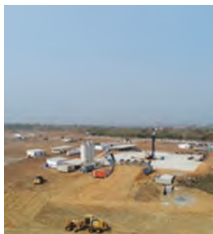
Sogea-Satom UK will source goods and services from the UK supply chain and boost UK exports to the region.
