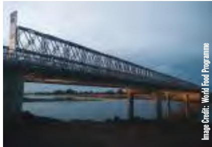
The Kwacjok Bridge is the latest WFP engineering project in South Sudan.
