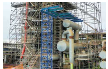
TG-60 supporting FlexBeam on site in Mpumalanga.
