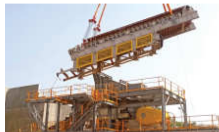
Crusher apron feeder first lift.
