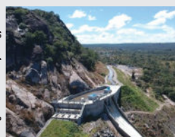
Achwa 2 hydropower project, 41MW, Uganda, developed and constructed by Berkeley Energy, with funding support from SEFA.
