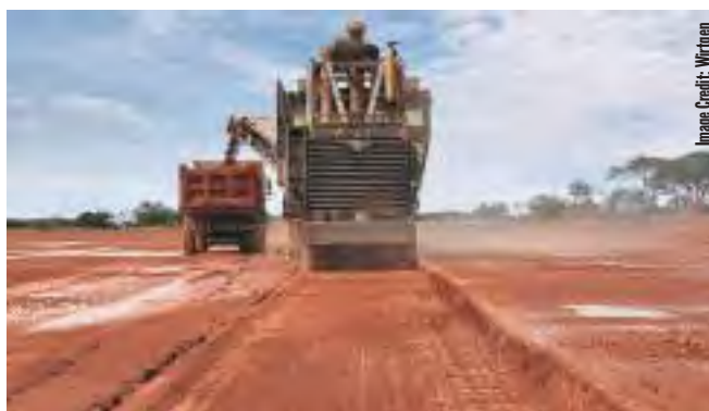
Wirtgen surface miners are used to open routes and develop the infrastructure.
