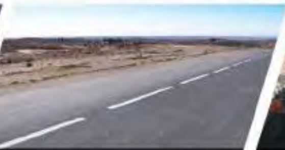
ZIMARA INFRA LINK • TOLL ROAD ZIMBABWE
