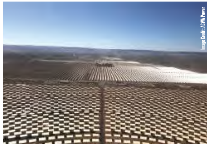
The Ouarzazate solar complex in Morocco is one of the largest concentrated solar plants in the world.
