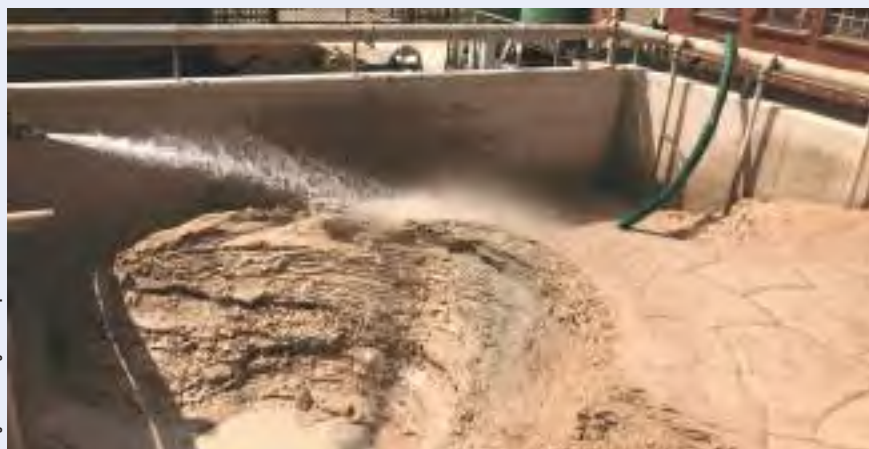
The team from Integrated Pump Rental used a hydro solution to clear the tanks of sediment.
