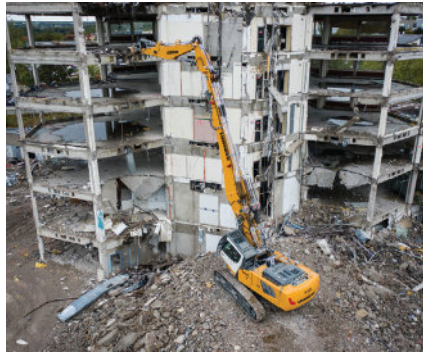
A new Liebherr crawler excavator: the R 940 Demolition replaces the R 944 C.
