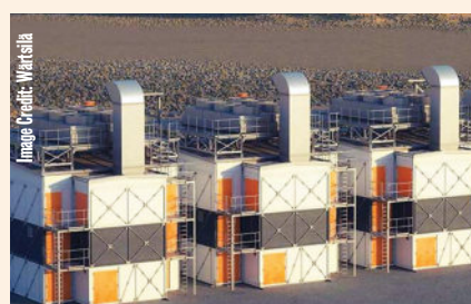
Four Wärtsilä Modular Block enclosures, each equipped with a Wärtsilä 32 engine are installed at the Syama mine.
