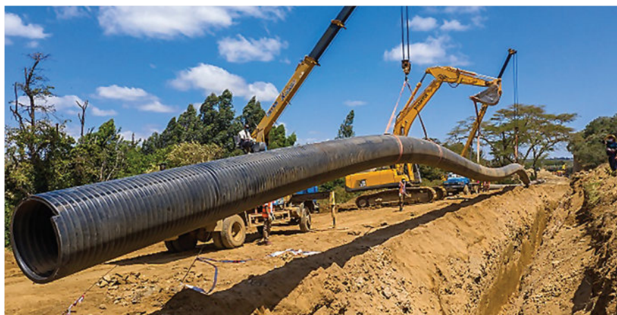
The installation of a Weholite pipe in Kenya.
