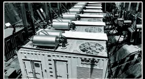
High Voltage 6.3MW Power Plant - Thailand
