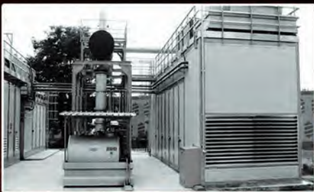
Bio Oil 2MW Power Plant - Italy
