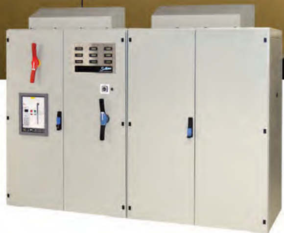
800kVA Sollatek AVR used on UK Grid Substations
