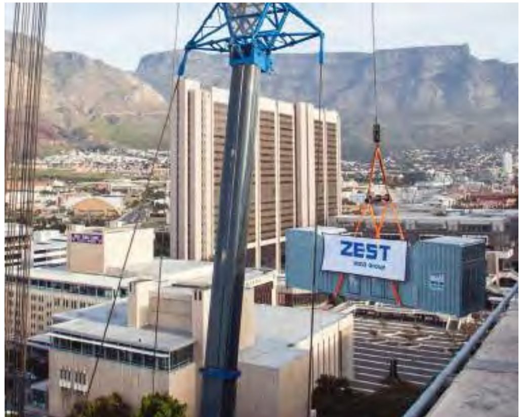
The lift of the Zest generator was done on a wind free day in Cape Town.
