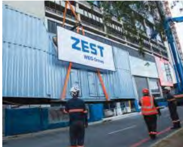
The 2000 kVA Zest generator during the initial stages of the generator lift.
