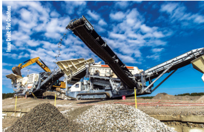
Metso mobile jaw crusher and scalping screen working on-site.
