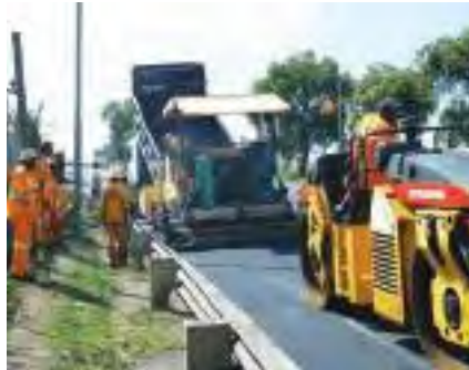
Application of EME asphalt by National Asphalt.
