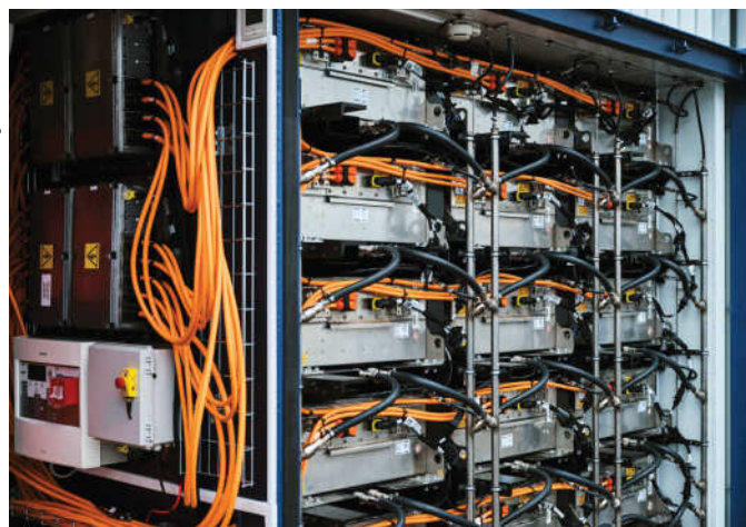
Volvo Penta's modular and scalable subsystem will be integrated into manufacturers' BESS applications.
