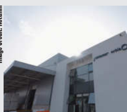
The manufacturing plant has officially opened in the Kenitra region of Morocco.
