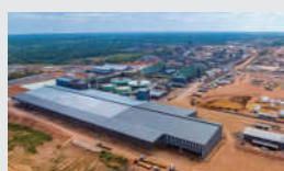
Kamo-Kakula’s concentrate storage and dispatch warehouse has been expanded to accommodate the larger production capacity.
