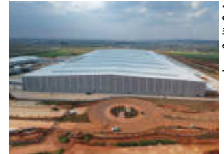
Image Credit: Genie The DSV Warehouse project's construction started in 2019.
