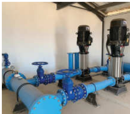
A Grundfos CR 125-5 pump installed in a water boosting application at a wine farm.
