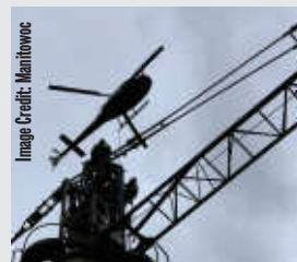
A helicopter lifts the components to assemble the Potain MCT 58.
