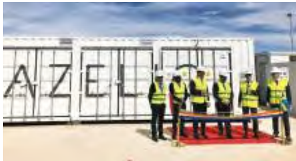
The renewable energy storage at the Noor Ouarzazate solar complex in Morocco.
