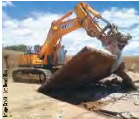
Image Credit: Jet Demolition Jet Demolition has the expertise to deal with complex heavy industrial demolition projects.
