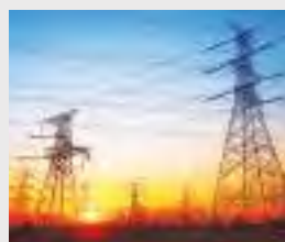
The new power line will establish Zimbabwe as a regional power hub. (Photo: zhengzaishuru/Shutterstock)
