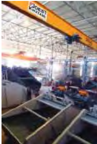
At Electra Mining Joest Kwatani will demonstrate the importance of on-site service in supporting its customers
