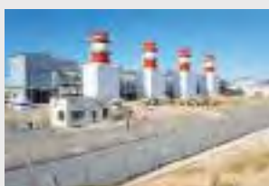
The Avon Peaking Power facility will provide much needed power and energy security
