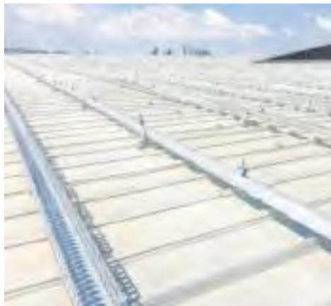
Lumax Energy has supplied a Renusol mounting system for ABB’s solar microgrid
