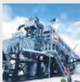
The product lines shown at Hillhead serve an increasingly diverse range of materials handling
