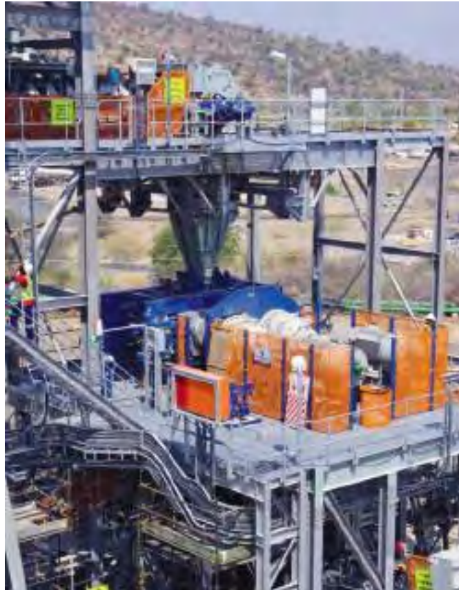
FLSmith’s will highlight innovations such as the high pressure grinding roller (HPGR) installation at Mogalakwena
