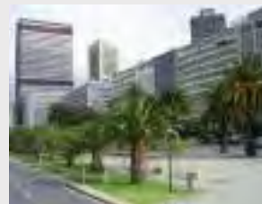
South Africa is a leader in green building (Photo: Joachim Huber/ Wiki Commons)
