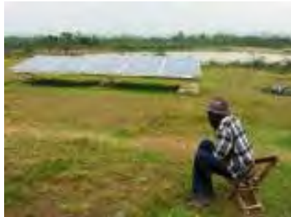
A solar mini-grid located in remote Masurura, northern Tanzania (Photo: Power Africa/Flickr)
