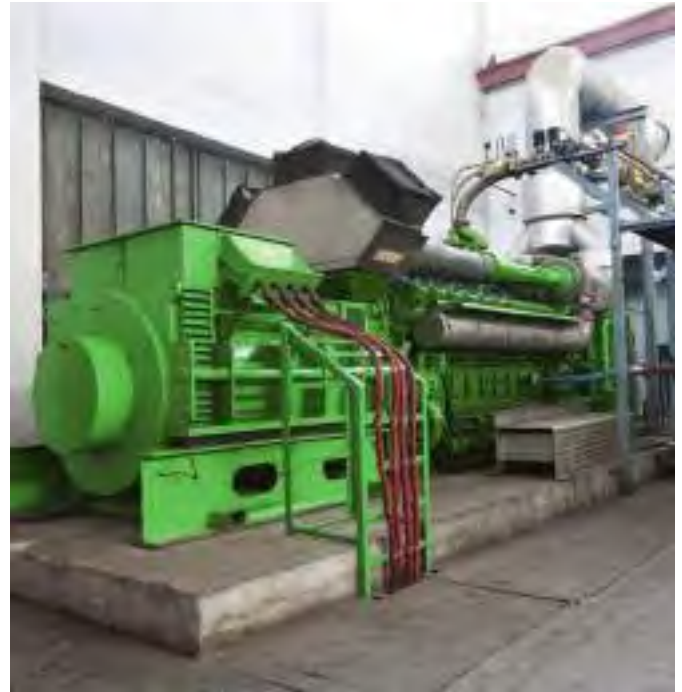
Gensets in textile factories like this may be a more common sight across the continent (Photo: Rehan Qureshi/shutterstock)
