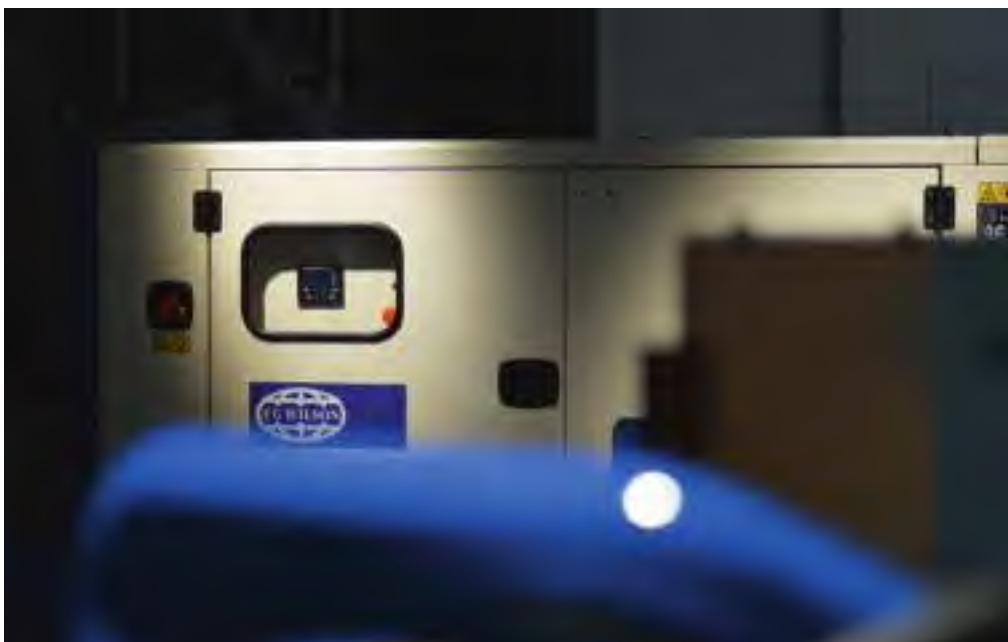
One of 600,000 FG Wilson’s generators installed since 1990 (Photo: FG Wilson)
