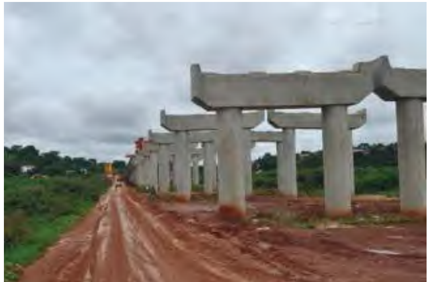
Section of the Kampala-Entebbe expressway. (Source: UNRA)
