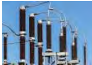
According to Camc, the project will be completed within 30 months. (Image: Chris Van Lennep Photo)
