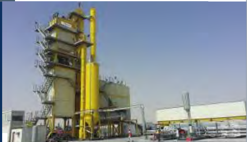
FAYAT MIXING PLANT
