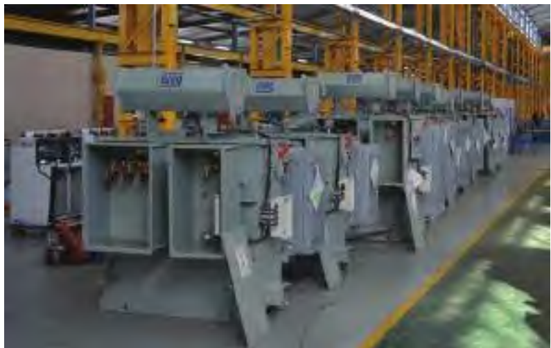
5 x 1 600 kVA 11 kV/433 V and 1 x 2 000 kVA 11 kV/720 V Transformers Export to Ghana
