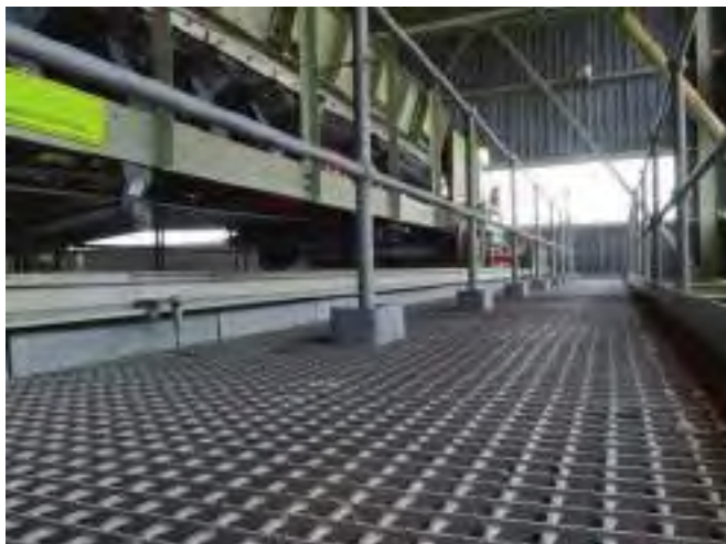
Rectagrid RS40 is used to create mezzanines, which optimises the use of previously dead space in a facility
