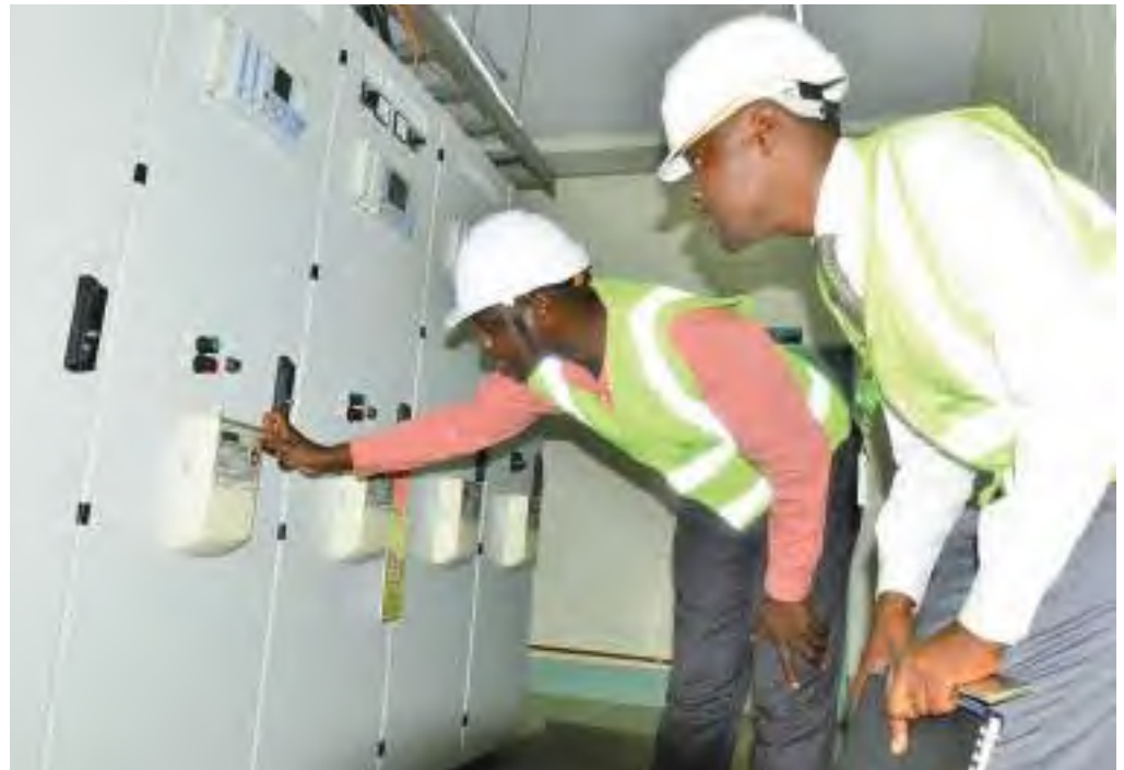
Engineers from Umeme, Uganda’s largest energy distributor, working at an electricity substation (Source: Umeme)
