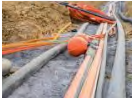
The new fibre optic plant in Durban is now operational (Source: Shutterstock ThomBal)
