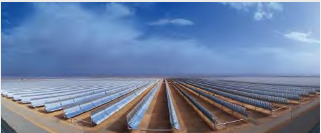
The first photovoltaic phase of the Noor solar plan (NOOR PV 1 programme) (Source: ACWA Power)
