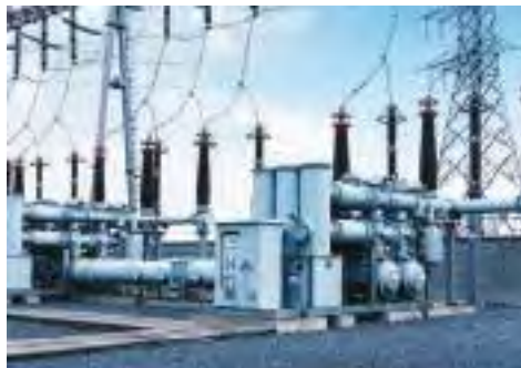
Kenya Power is looking to buy locally assembled transformers during the 2016/17 financial year (Source: Shutterstock gyn9037)
