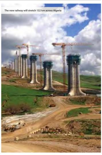
petal' shape, the piers required the design of customized steel formwork panels for the outside, while, for the inside, Doka's largearea formwork Top 50 was used. In total, 16 SKE50 and 4 SKE100, plus climbing units, supported the 4.5 m tall wall formwork.
