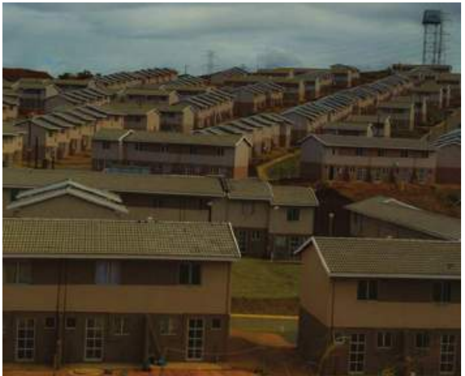
The first 482 houses in the initial phase at Cornubia have been finished and handed over to residents (Image: GCIS)
