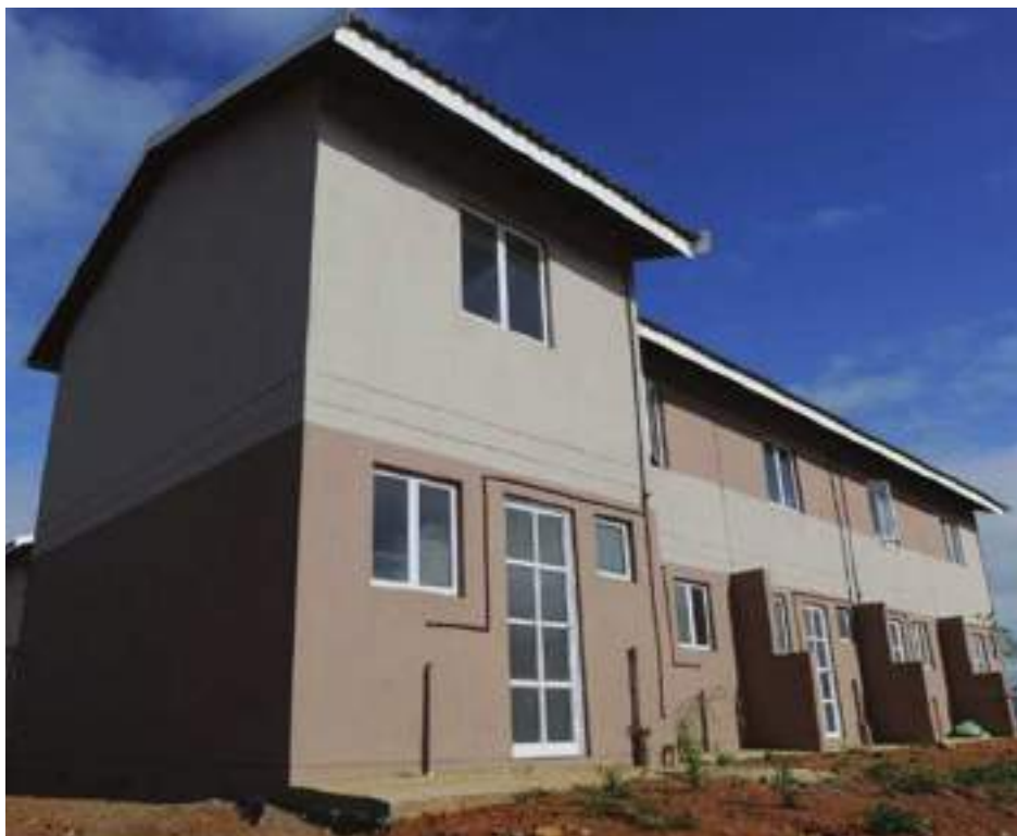
There is a strong focus on ensuring the delivery of affordable housing in sustainable and habitable settlements (Image: GCIS)
