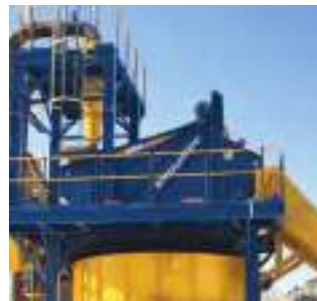
Enduron screen being installed in a quarrying application
