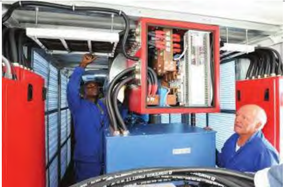
A view inside a containerised generator set from Zest WEG Group's Generator Set Division
