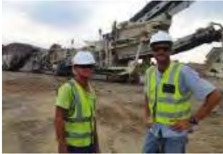
B&E International is crushing aggregates for use in the reconstruction of the Maputo airport runway
