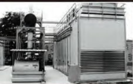
Bio Oil 2MW Power Plant - Italy
