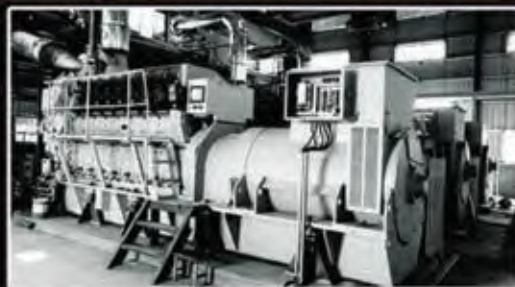
Yoboki-Lac Assal HFO 4.8MW Power Plant - Djibouti
