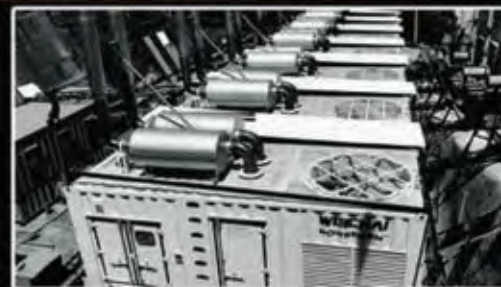
High Voltage 6.3MW Power Plant - Thailand
