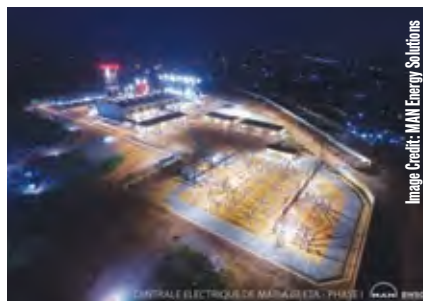
The Maria Gleta power plant will supply the grid of Benin with 127MW of electrical output.
