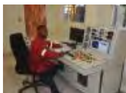
100 MVA 132 kV Testing Bay
