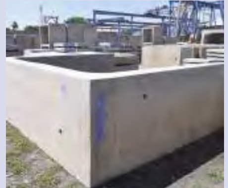
Chryso will supply 20 admixtures for use in self-compacting concrete
