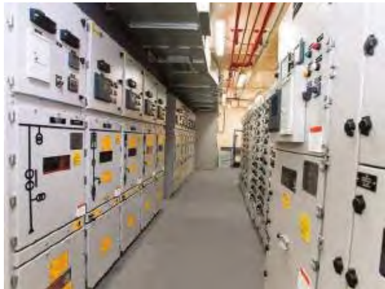
LV and MV Switchboards inside "E" House
