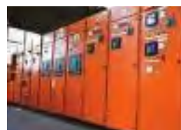
SC100 Motor Control Centre
