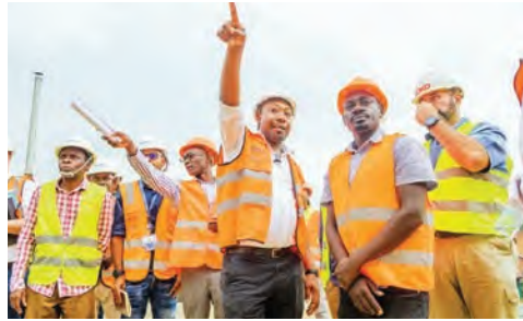
James Byaruhanga with other project members at the Raxio Data Centre construction site in Namanve.
