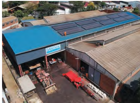
Solar power is driving Sandvik's mining and rock technology facility in Zimbabwe.
