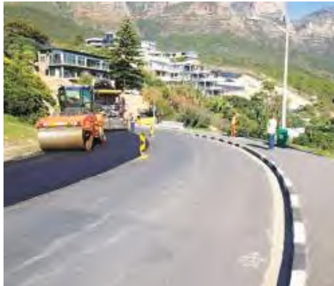
Cold recycling technologies for reclaimed asphalt were used along Camps Bay Drive.
